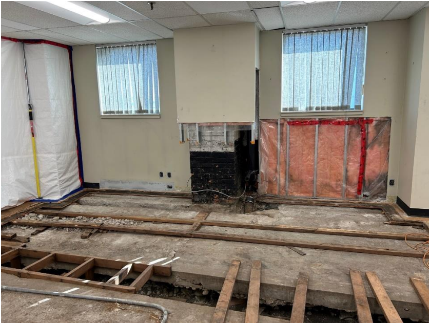
Pictures of the construction at the club house.
